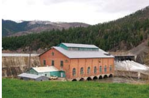
Last Look. Milltown powerhouse and dam will be removed in the dry.
