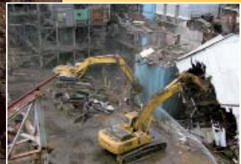
DEMOLITION, DECONTAMINATION & DECOMMISSIONING
