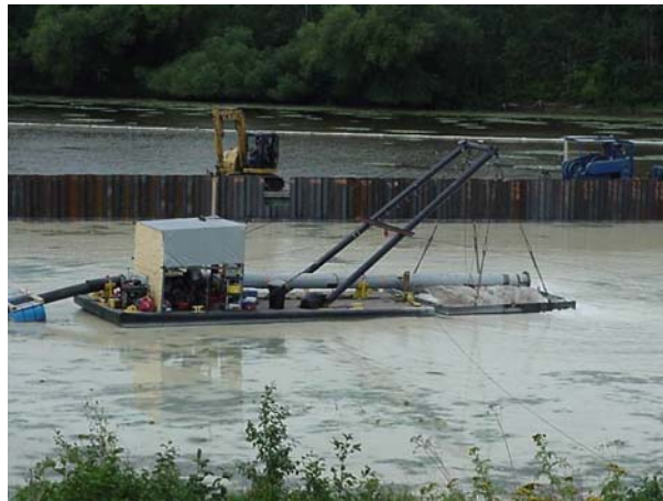
Figure 1. Sub-capping operations
