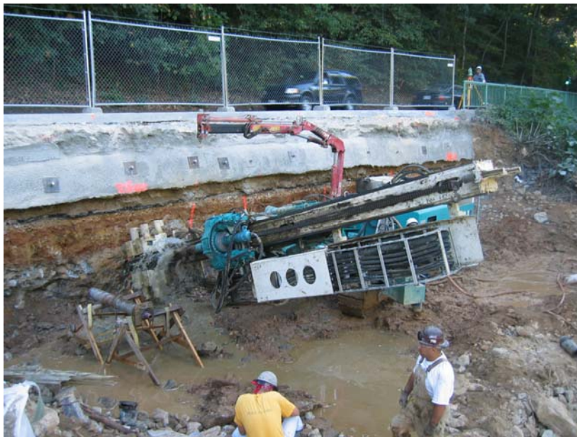
Figure 9 - Soil Nail Installation Showing Old Pavements, Rubble and Soil Fill
