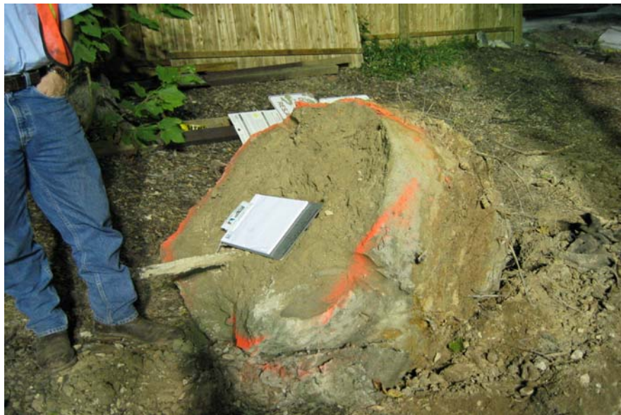
Figure 7 - Excavated Jet Grout Column Partially Removed From the Ground
