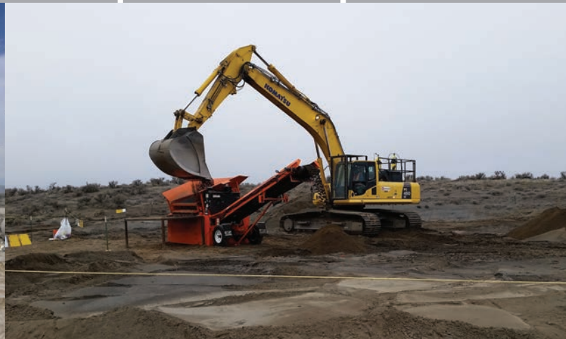
Hanford Management of Munitions & Explosives of Concern (MEC), Richland, WA. MEC removal and disposal at a 125 acre former firing range.
